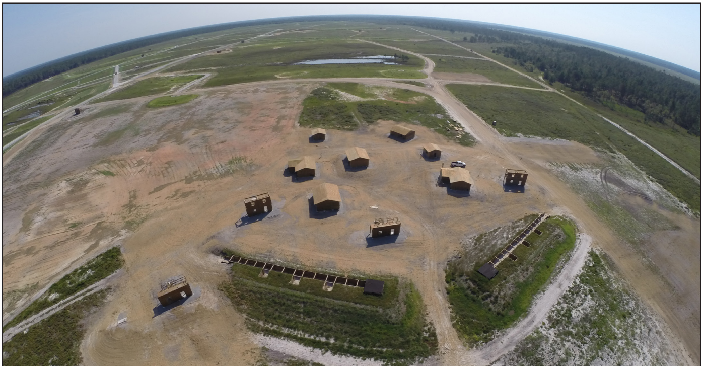
An urban building cluster and trench objective on the Multipurpose Training Range at Fort Stewart, Georgia.
